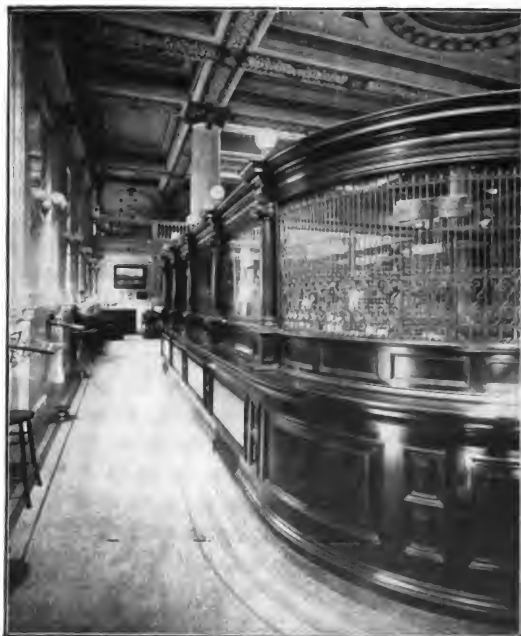
VIEW OF PORTION OF BANKING ROOM, CORN EXCHANGE NATIONAL BANK, PHILADELPHIA.
